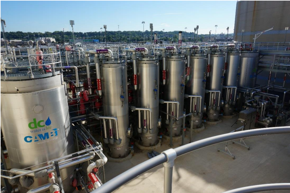
Figure 40: Thermal Hydrolysis Process plant at DC Water's Blue Plains WWTP, Washington DC
