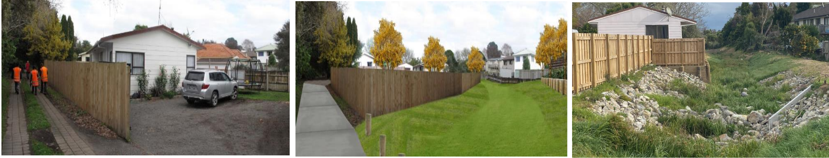
Above Left) Prior to work Above Middle) Schematic Above Right) Overland flowpath nearing completion – looking from driveway to 36E Meadowland Street to Matua Saltmarsh
