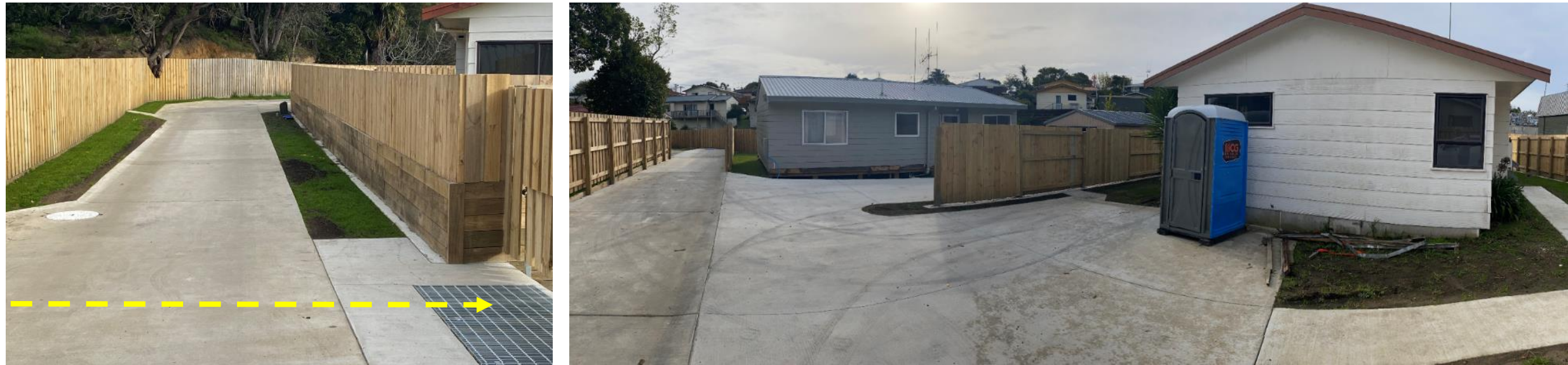
Above Left) Completed driveway/fencing leading to 36E Meadowland Street – yellow dash is direction of overland flow discharging via grate to swale Above Right and Below Left) 3x properties relocated out of swale footprint. To be refurbished and sold as freehold sites.
