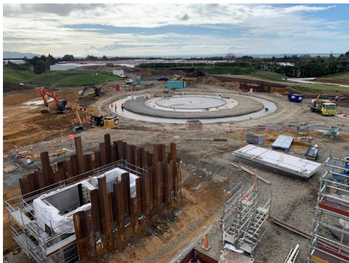
Photo of the reservoir platform at the Waiāri WTP site, with the sludge thickener balance tanks in the foreground.
