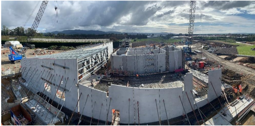
Photo of the construction of the Waiari WTP membrane machine hall and clarifier.
