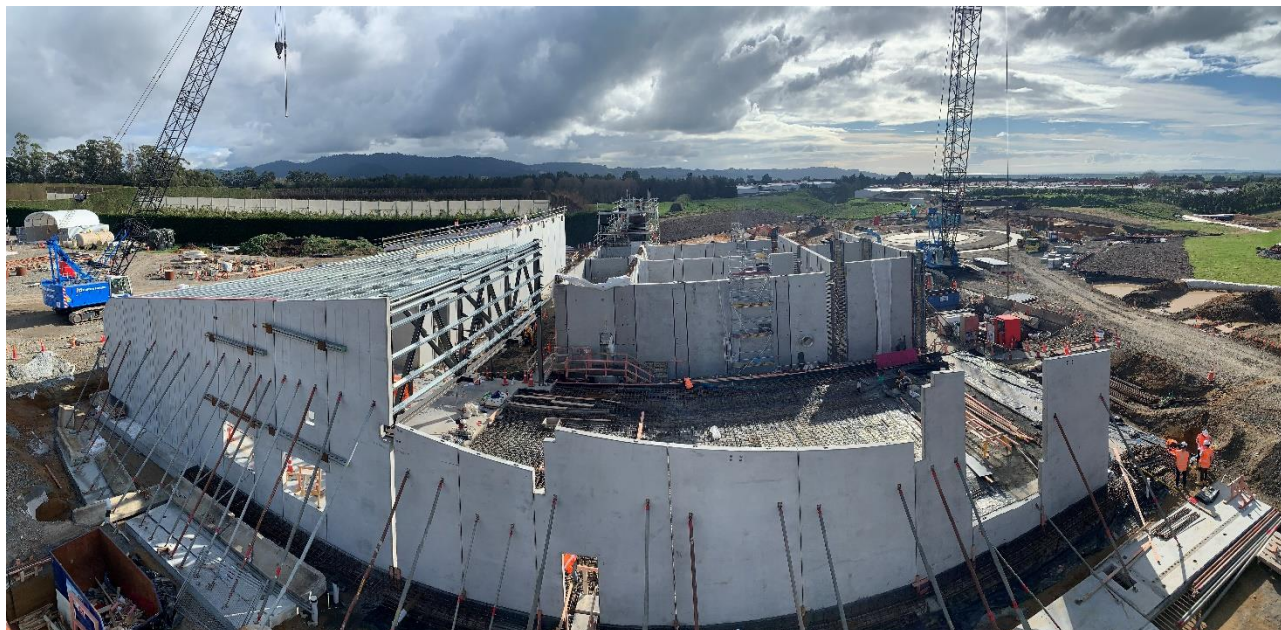
Recent photo of the water treatment plant construction site
