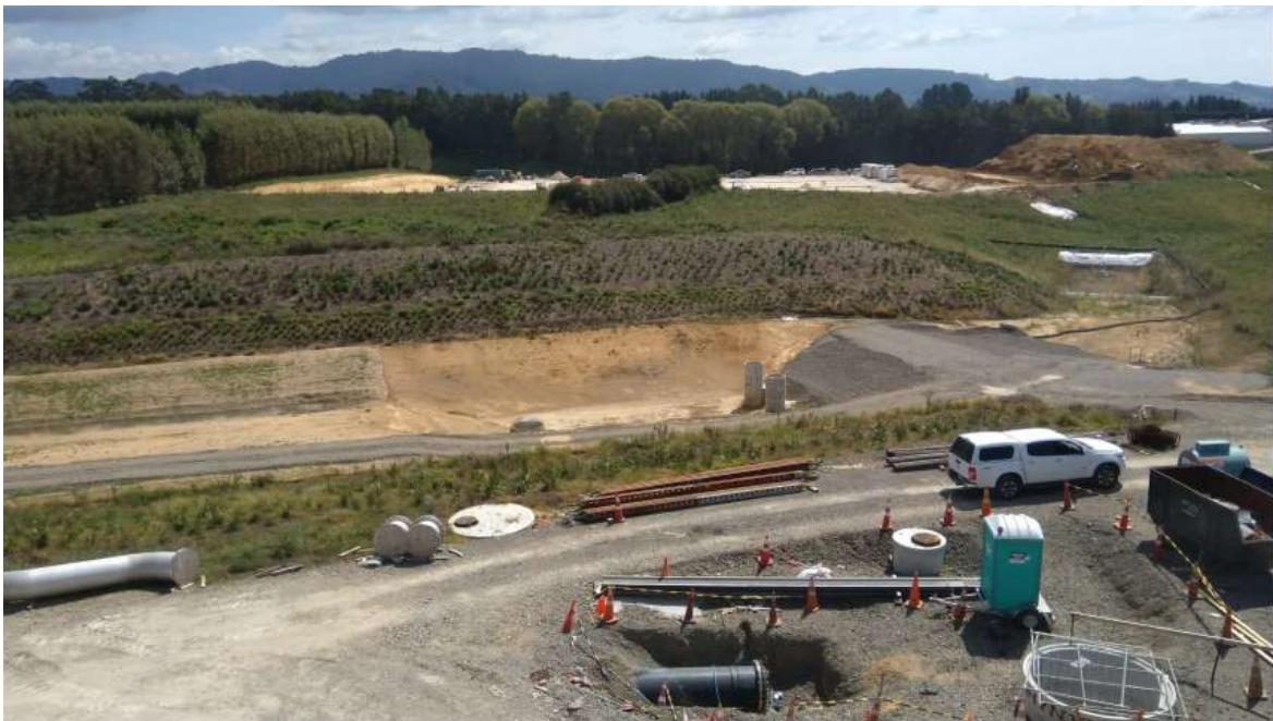
WTP permanent stormwater detention and treatment pond nearing completion
