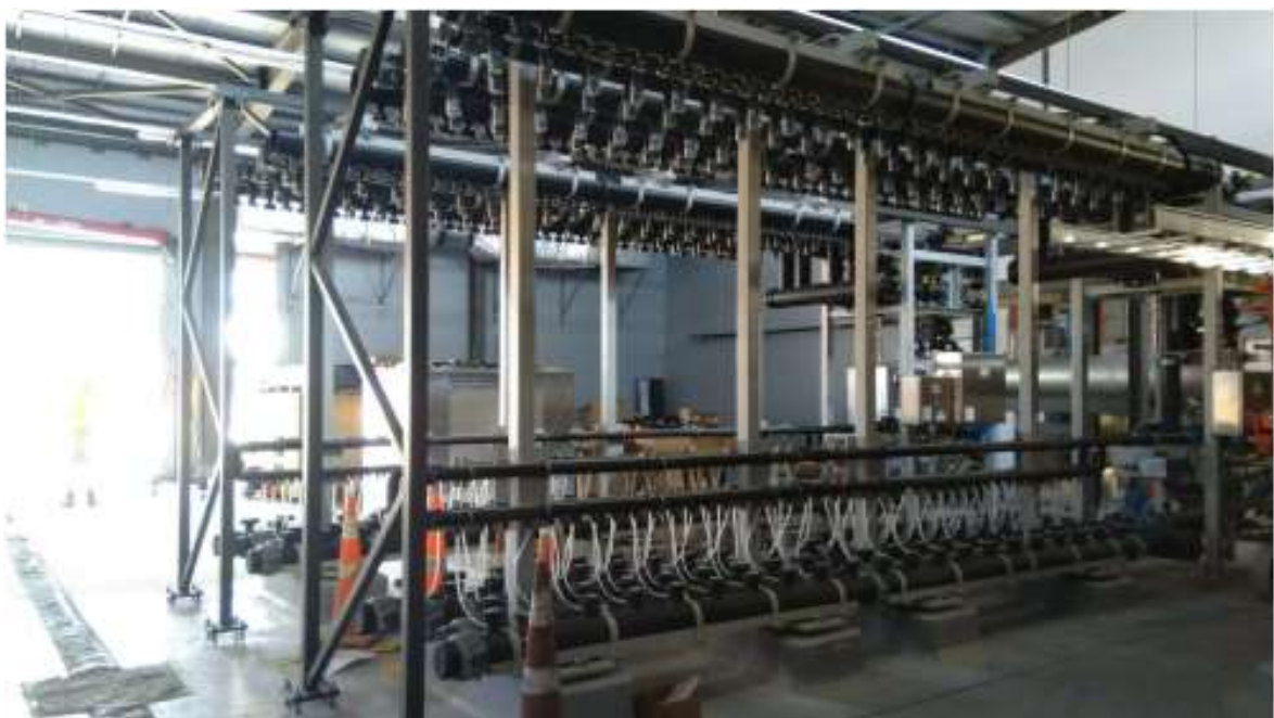
Membrane Hall: Skids ready for the microfiltration membrane units to be installed
