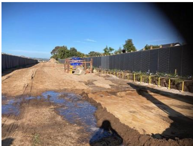
Dewatering installation prior to trenching.
