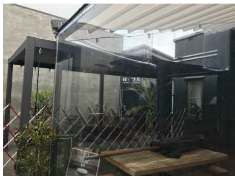
Full clear screens and new retractable louvre system
