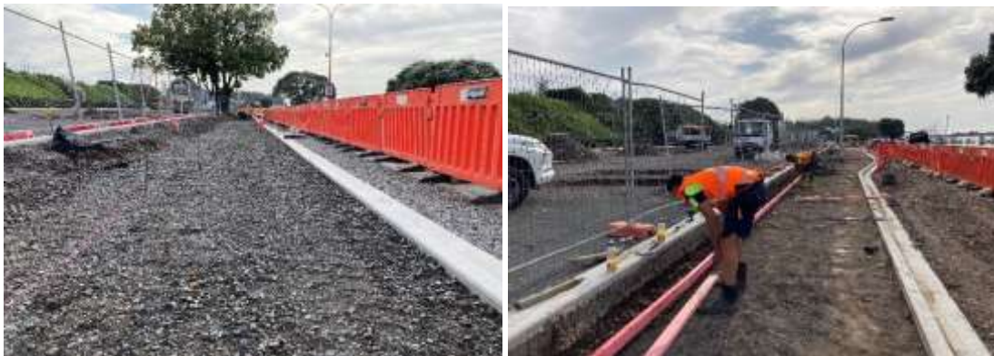
Dive Crescent – area/footpath prepared, compacted fill now completed.
