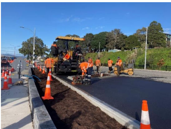
Crossroads commence the laying of bitumen.
