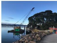
In preparation for the development of a new structure at Beacon Wharf the removal of the current wharf, an unstable structure, was needed. Most of the demolition work required to dismantle the wharf is being executed from a barge, necessitating careful planning and the implementation of specific safety measures. A temporary works design has been crafted to address the lifting requirements of the demolition process while ensuring the safety of the workers operating from the barge.
