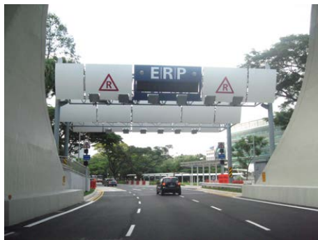
Figure 12 Singapore ERP gantry
