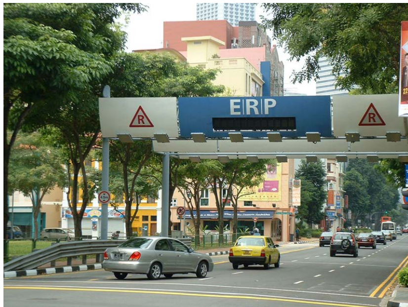
Figure 16 Singapore ERP gantry
