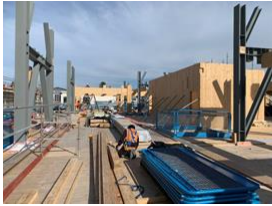
Structural steel bracing frames and timber structure for level 3 progressing.
