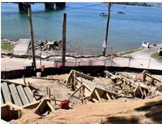
The concrete pour for the bottom section of the stairs has been completed.
