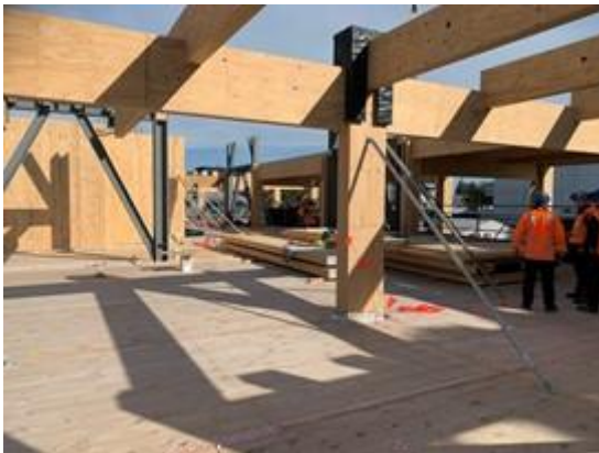
These timber structure beams and columns will be visible to those working in 90 Devonport Road.
