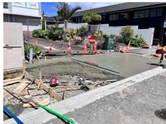
Driveway concreting works on the southern side of Elizabeth St East.
