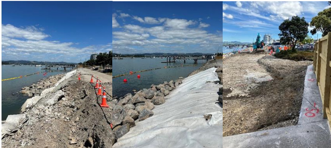
Construction of the seawall, footpath, boardwalk and gardens.
