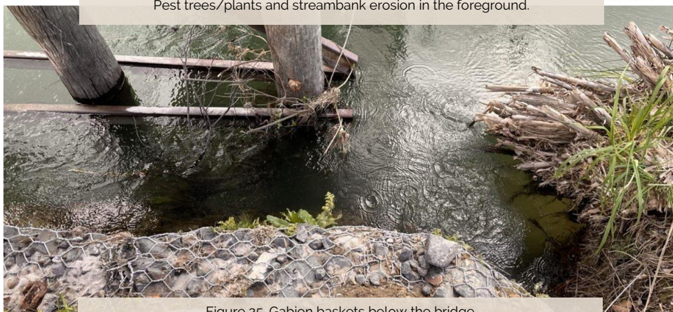
Figure 25. Gabion baskets below the bridge
