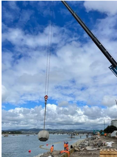
Installation of the living seawall units, pods at low tide, and then at almost high tide
