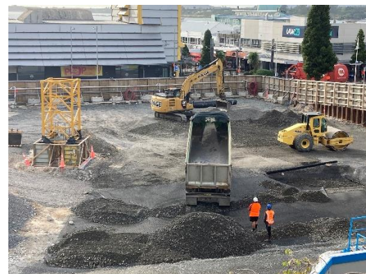
600mm-thick load bearing platform.
