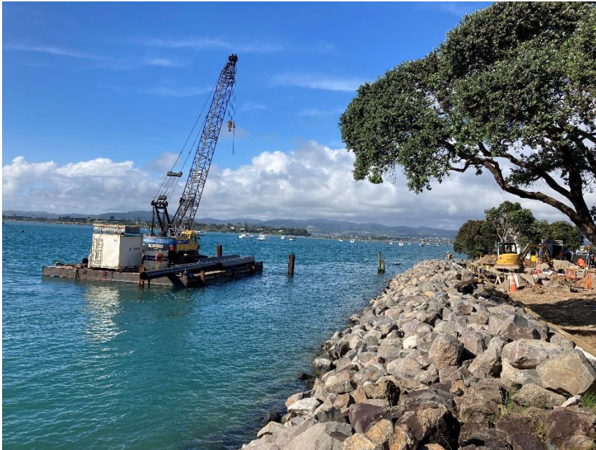
Piler barge set up at the Beacon Wharf.
