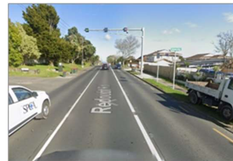
Tidal Flow example, Redoubt Rd, Auckland
