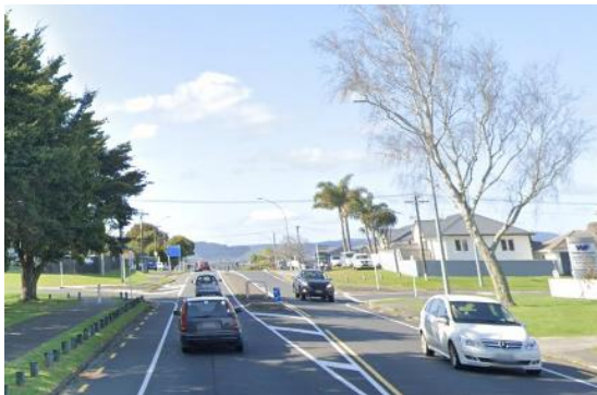
Fifteenth Avenue currently between Cameron Rd and Devonport Rd
