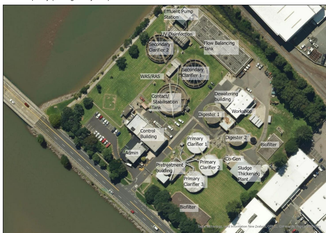
Figure 3. Aerial view of the Chapel Street wastewater treatment plant with components labelled
