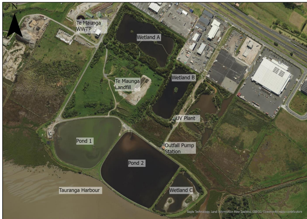
Figure 5. Aerial image of Te Maunga treatment ponds, wetland, outfall PS and UV plant.
