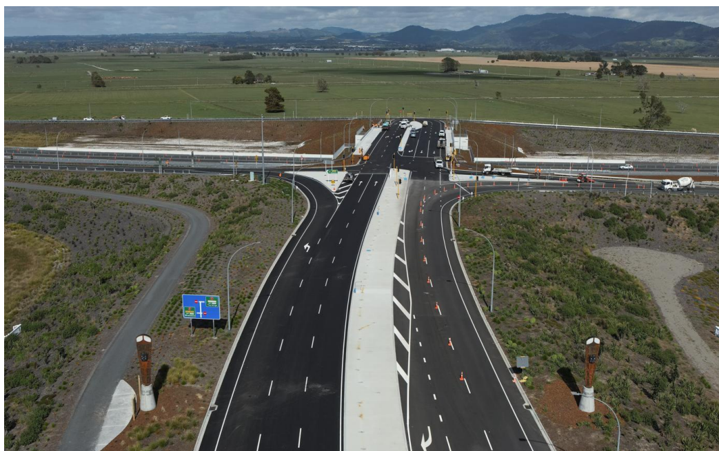
Pāpāmoa East Interchange – aerial perspective from The Sands Ave towards the new overbridge
