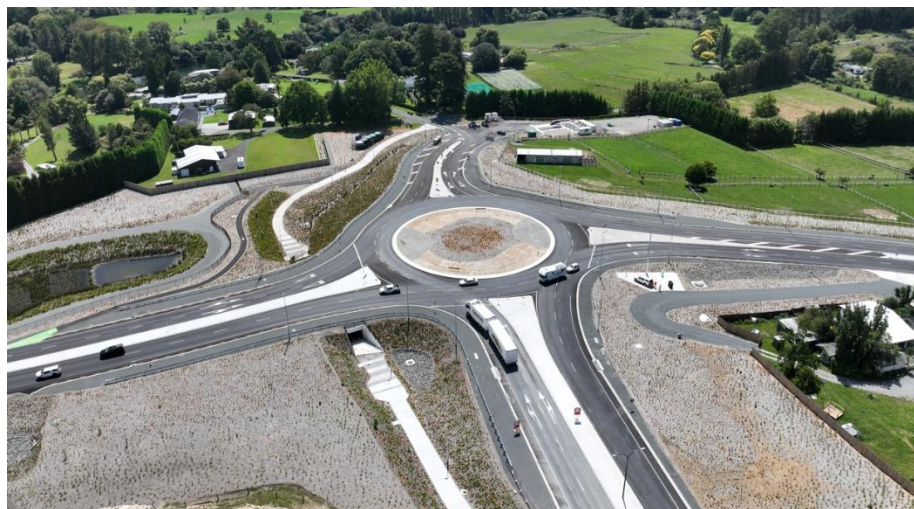
SH29 / Kaweroa Drive / Redwood Lane Roundabout - Complete
