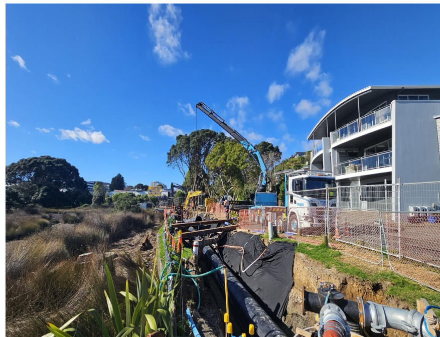
Churchill Foreshore Sewer (3rd Ave section)
