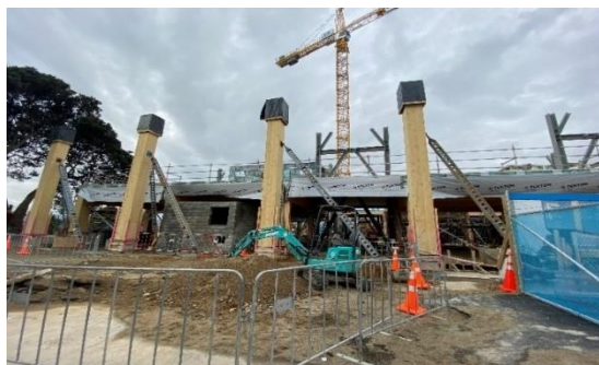
Structural steel K frames installed for level 2
