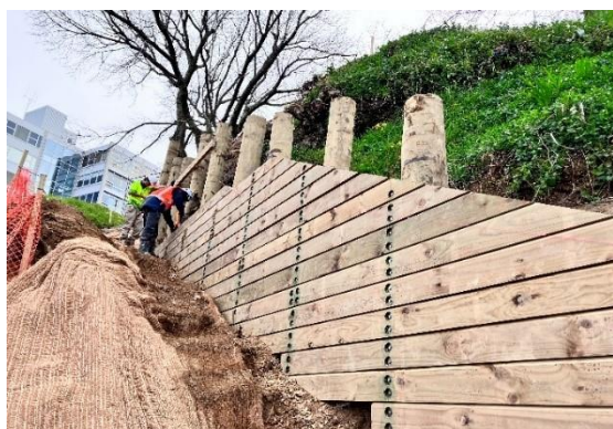
Lagging works for retaining wall one
