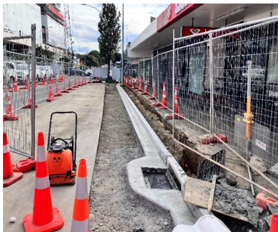
Kerbing install completed on the northern side of Elizabeth Street East
