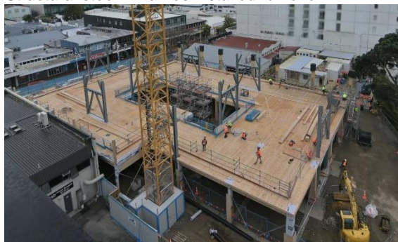
First floor CLT complete. LTMcG targeting 1 floor completed per month
