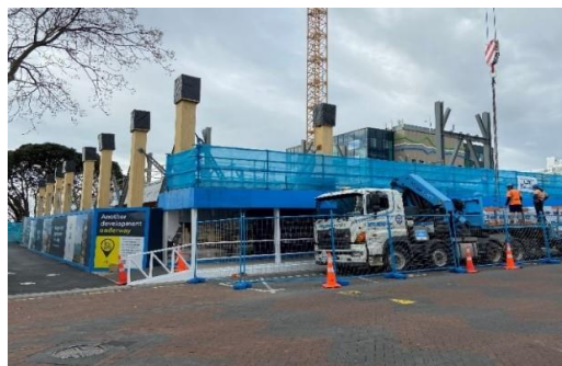
Structural CLT timber for second level being unloaded
