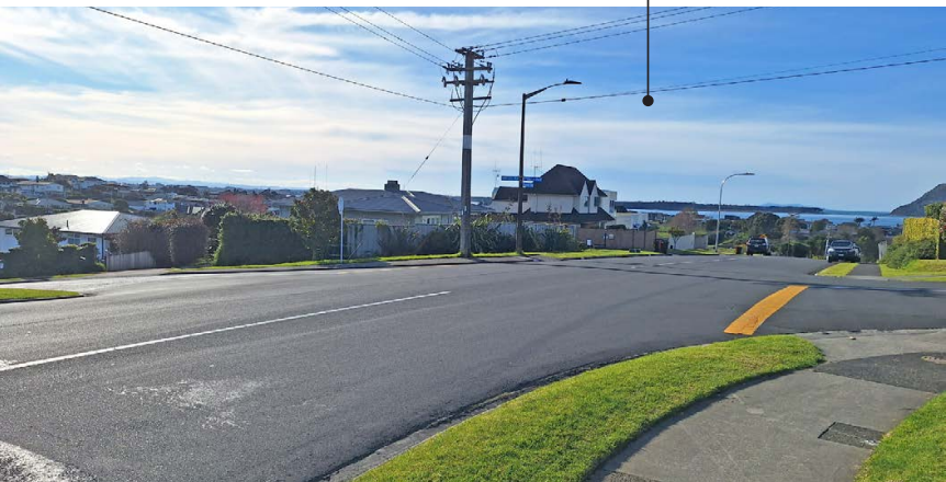
Hinewa Road / Grange Road Intersection, wide carriageway, difficult sightlines due to slope and speed of traffic makes it hard to cross safely
