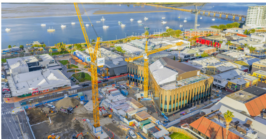
Civic Precinct under construction
