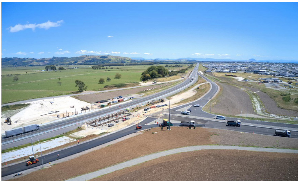
Pāpāmoa East Interchange under construction
