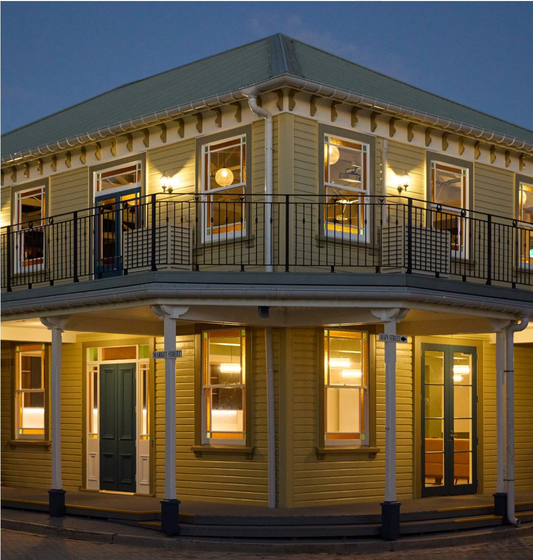
Photo: Historic Village. Photo credit: Hunter Studios
