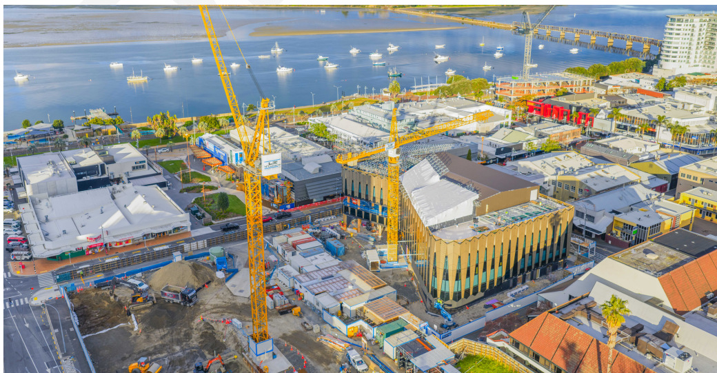
Civic Precinct under construction
