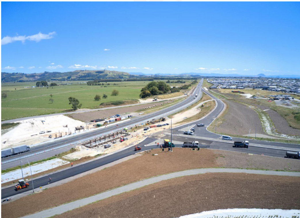
Pāpāmoa East Interchange under construction
