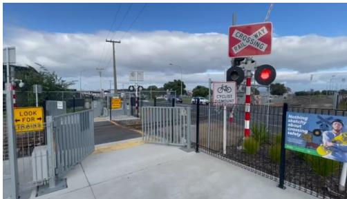
Signalisation of Rail Crossing at Hull Road
