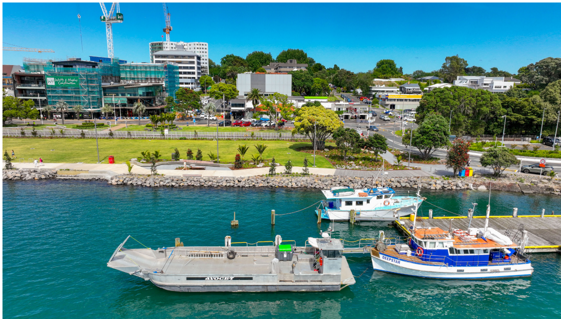
Upgrading of the seawall at The Strand. Tauranga City Council
