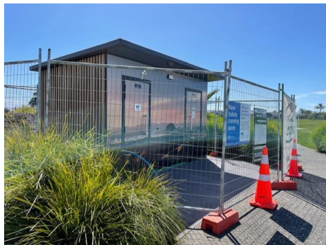
New Toilet Facility in Monticola Reserve, Papamoa
