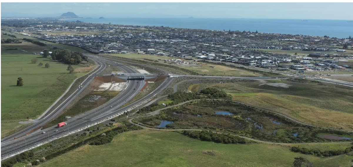
Pāpāmoa East Interchange – aerial perspective from east of the new interchange
